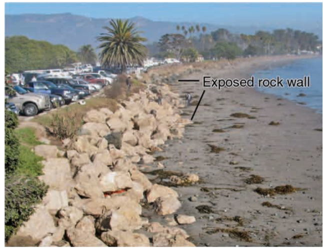
Fig. 5.17b. High waves in early December of 2007 caused erosion of the hot spot, exposing the rock wall.
