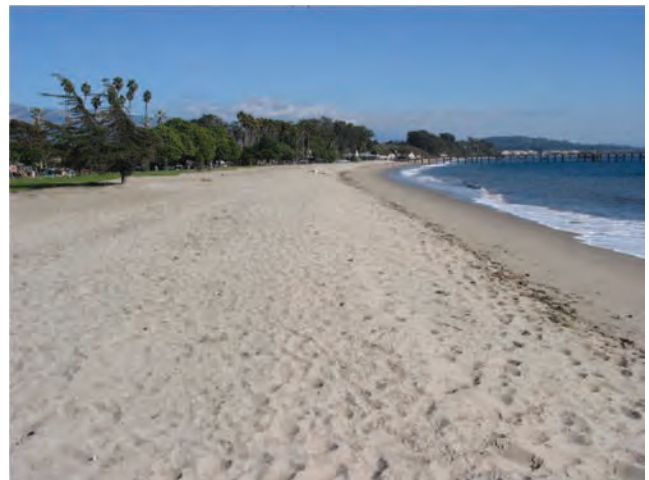
Fig. 5.19b. Goleta Beach following beach nourishment, summer 2005. Rock sea wall is buried below the sand.
