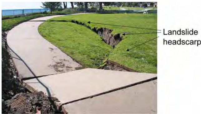
Fig. 2.17a. Small landslide on sea cliff above Shoreline Park that occurred in late January 2008. The curved headscarp is the landward limit of the slide. Another headscarp is present in the sea cliff. Similar older slides are common at the park, forming the wavy top of the cliff.
