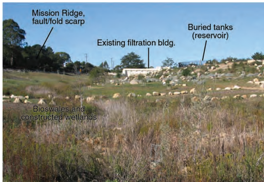
Fig. 6.2. Sheffield Reservoir. Once an open reservoir to store water is now a park designed as a natural area. Huge tanks now store the water. Filtered water is delivered to city users, 2007.
