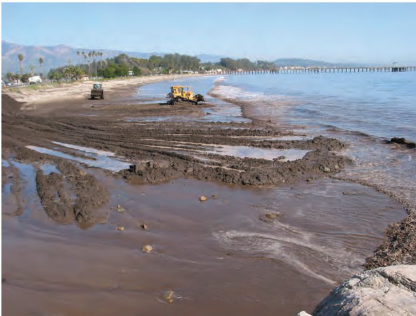
Fig. 6.27. New beach nourishment at Goleta Beach in 2010. The supply of sand was from sediment control basins on local streams that filled with sediment following the Jesusita Fire in 2009.
