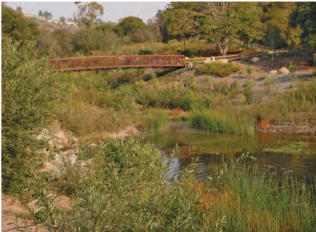
Fig. 3.11b. Restoration of Mesa Creek included opening the creek from a covered culvert, removal of introduced species of plants, and planting of native plants, 2007
