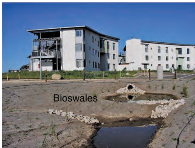
Fig. 5.11b. Manzanita Village student housing, 2003. Bioswales had just been constructed.
