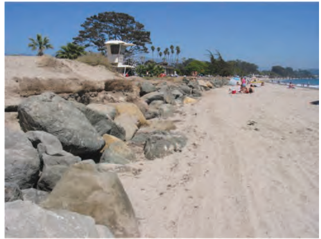
Fig. 5.19a. Rock sea wall, constructed in 2003 following erosion at Goleta Beach.
